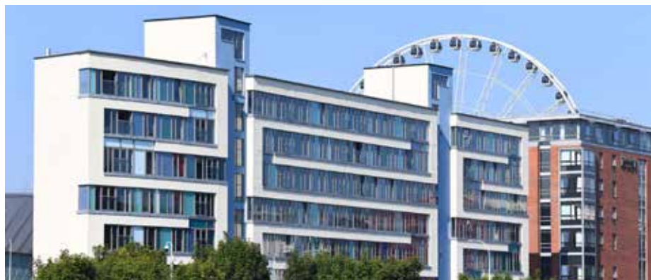
Dockside Aparthotel: the property saw an approximate 75% recovery in the original indebtedness position from a base position of negligible value. Image courtesy of Fletcher Bond
